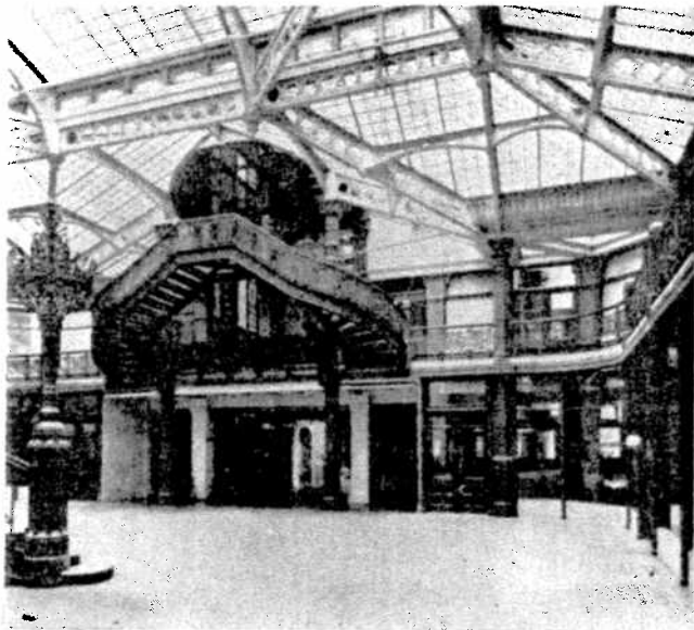
Skylit court lobby as designed by Root.
